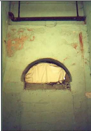
Blocked window and beam socket above.
