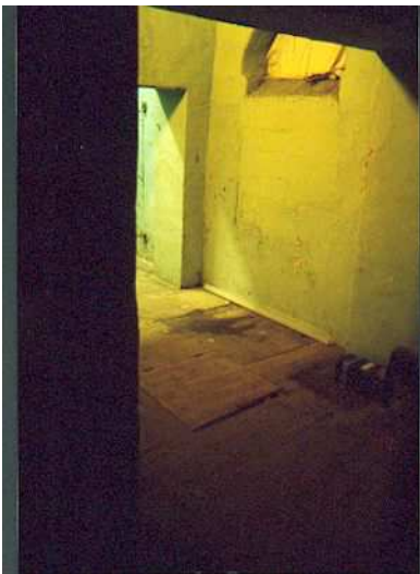
View into execution chamber from witnesses' doorway.
