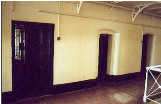
Another view of condemned cell, with corridor to gallows to left.
